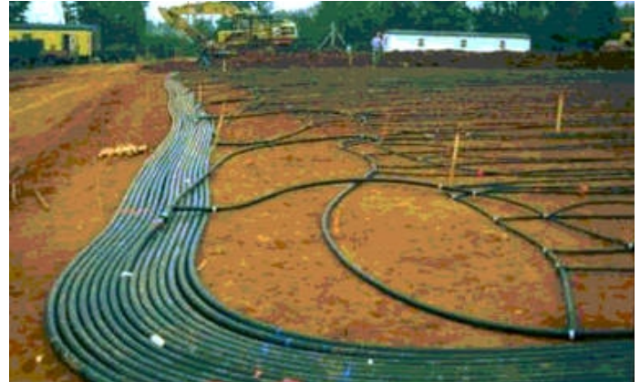
A view of a ground source heat pump used for heating and cooling a home. Photo courtesy of NRCAN
